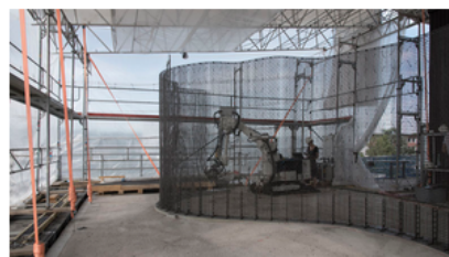
Mesh Mould and In situ Fabricator, 2016-2017 in the DFAB HOUSE
