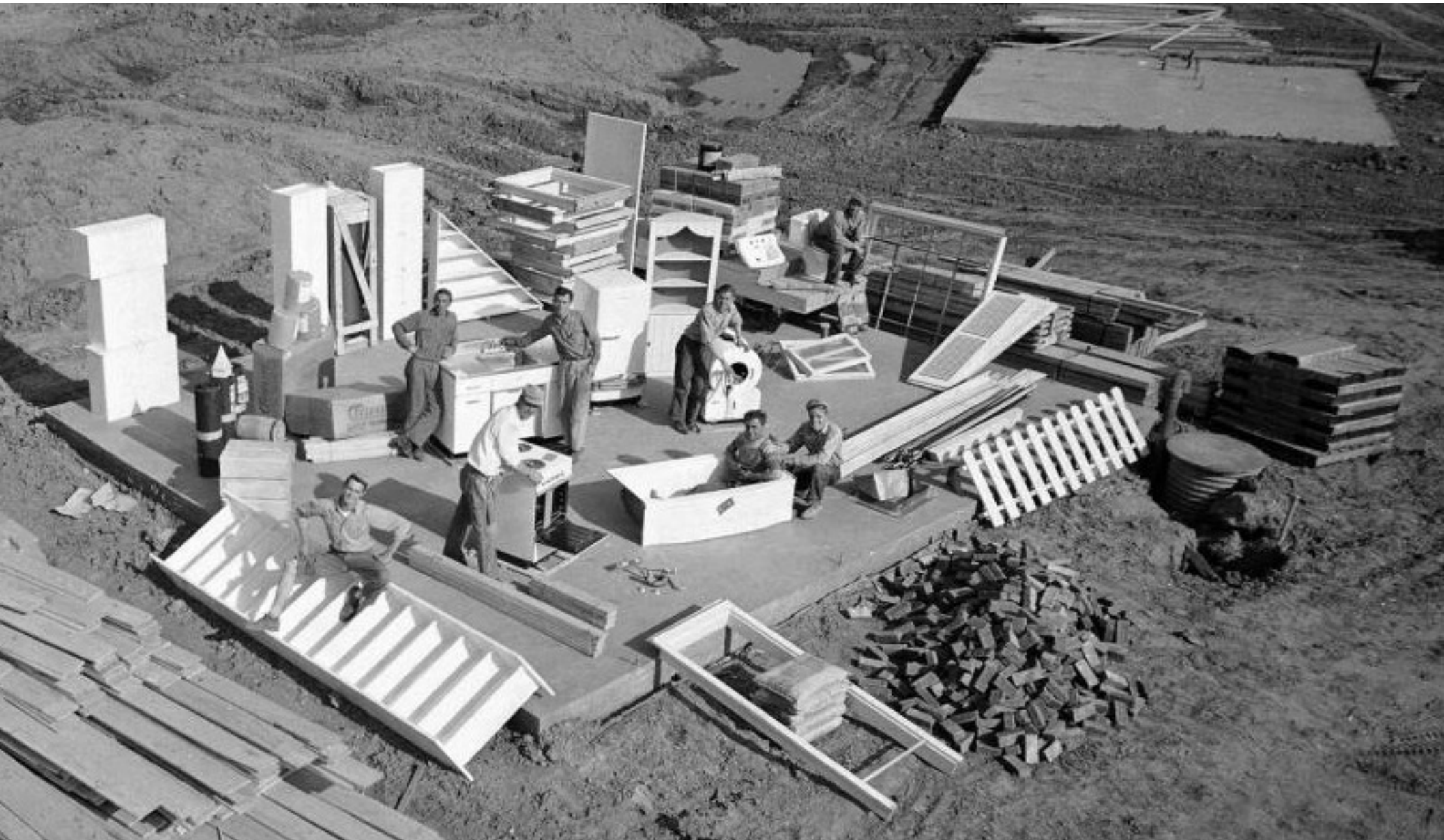
Tony Linck, for Life magazine, Workmen and the materials to construct a house gathered in a lot before construction, June, 1948
