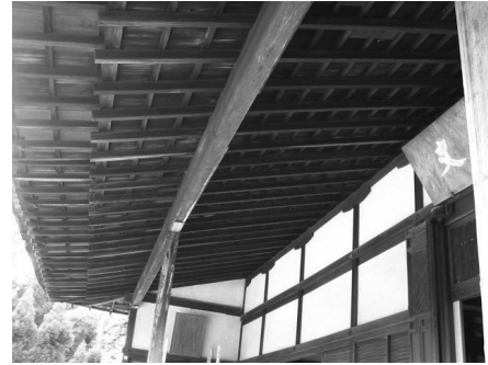
Fig.20. The southern eaves of the temple at Ryôanji with light-coloured wooden rafters. (Photo: Jose M. Cabeza)
